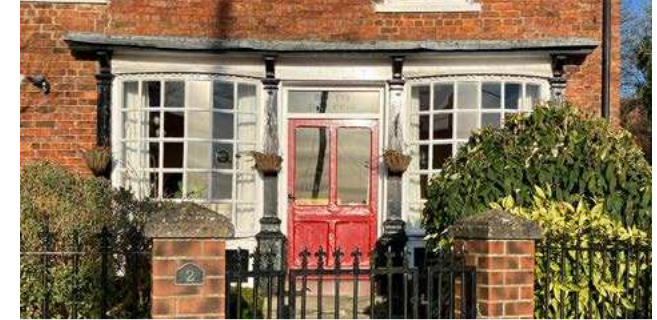
Figure 33: The Post Office (Grade II Listed). Brick with gabled slate roof and stacks. Two bay shopfront supported by wooden pilasters.
