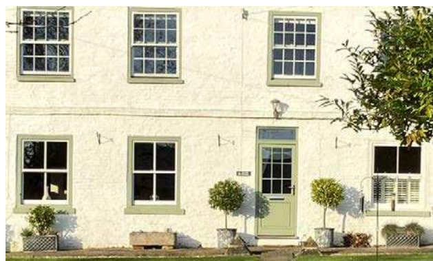
Figure 80: Light painted brick.
