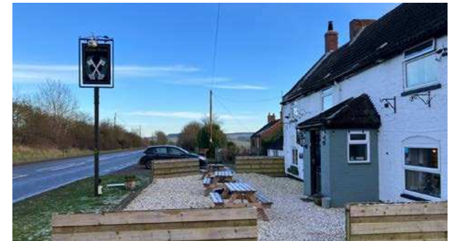
Figure 16: The Cross Keys Inn in Grasby is a key amenity for the neighbourhood area.
