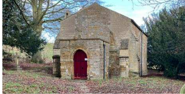
Figure 30: The Church of All Hallows (Grade II* Listed). Limestone, ironstone, slate roof tiles and brick blocking.
