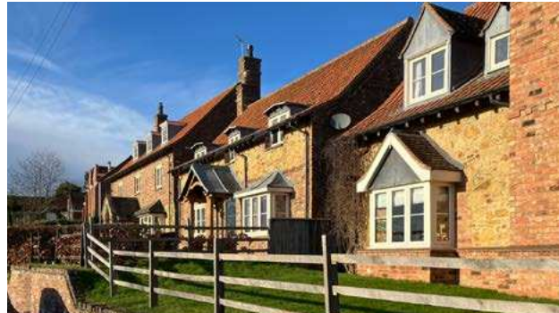
Figure 44: Detached houses in Grasby incorporating red brick and ironstone features.
