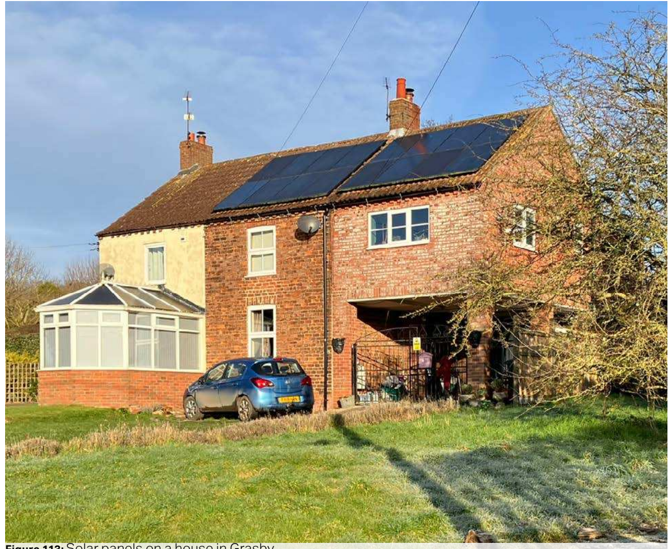
Figure 113: Solar panels on a house in Grasby.
