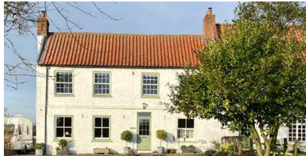
Figure 31: The Old Vicarage (Grasby) (Grade II Listed). Painted brick and red clay pantiles. Plain sash windows and chimney stacks.
