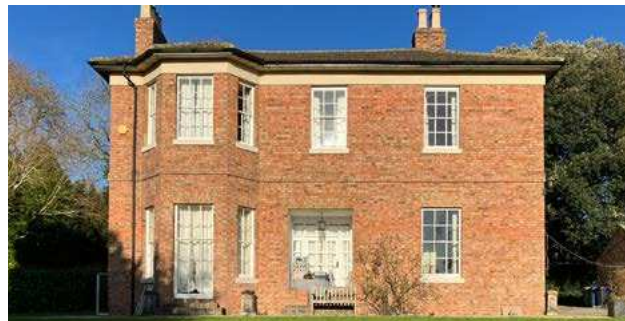
Figure 32: The Grange (Grade II Listed). Brick with three brick chimney stacks. Plain sash and canted bay windows.
