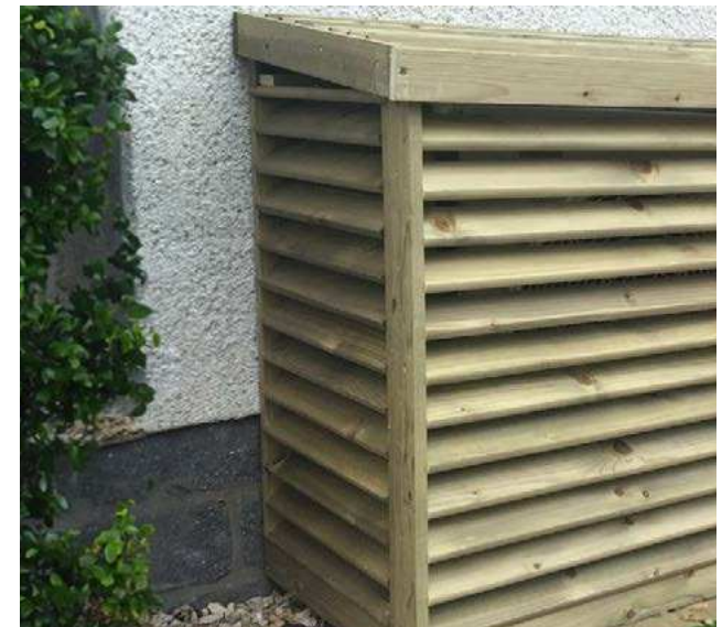
Figure 117: Air source heat pump housing covers the unit and harmonises with the building aesthetic.
