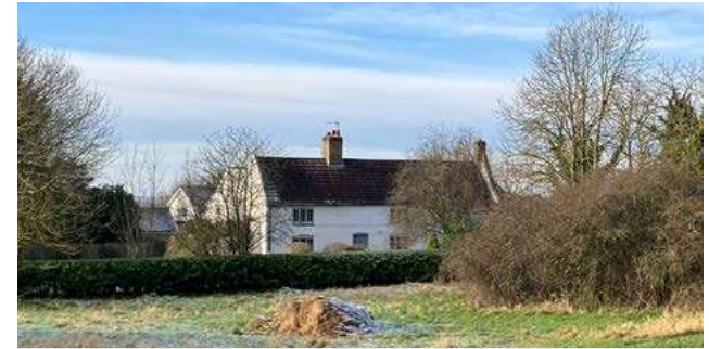
Figure 40: Island Cottage (Grade II Listed). Rendered brick with raised brick coped gables and kneelers, axial ridge stack and one gable stack.
