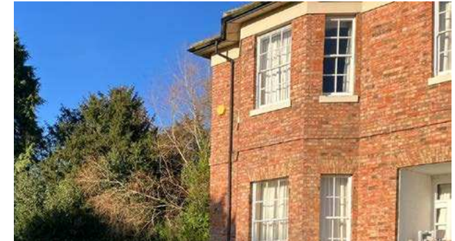
Figure 89: Two storey canted bay windows on the Grange in Grasby.
