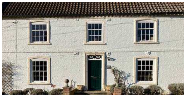
Figure 38: Tithe House (Grade II Listed). Colour washed brick, pantiled roof with stone coped gables and kneelers and sash windows.
