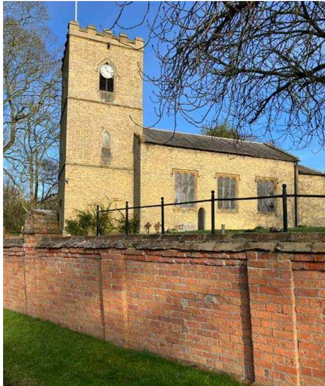
Figure 35: The Church of Saint Nicholas (Grade II Listed). Yellow brick, ashlar dressings, slate roof with lead dressings.
