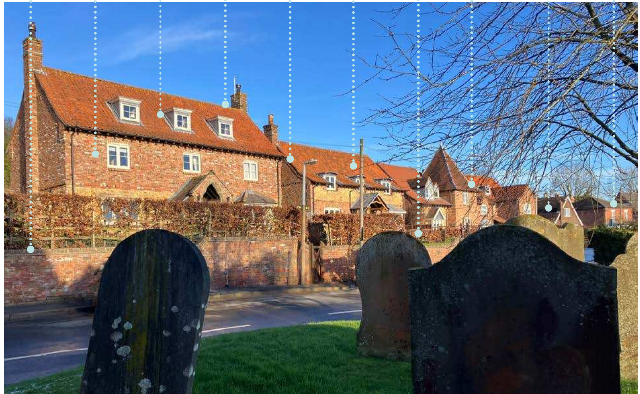
Figure 109: Development on Vicarage Lane of a scale, mass, density, height and level of set-back that responds to its historic neighbours and has a positive effect on the area's overall character.
