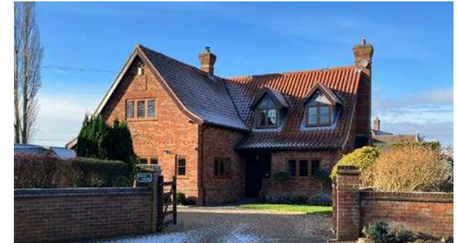
Figure 47: A 20th Century house in Searby with steep pitched pantile roofing and chimney stacks.
