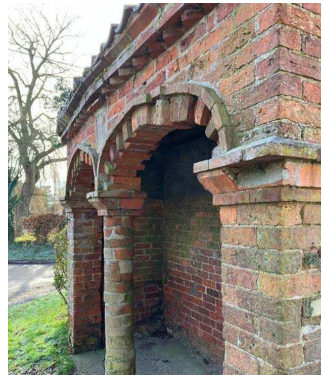
Figure 41: Roadside shelter. Grade II Listed. Red brick, pantiled gabled roof, two 4-centred brick arches supported by central round brick pillar.
