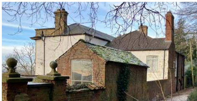
Figure 36: Owmy Mount (Grade II Listed). Yellow brick, ashlar dressings, hipped slate roof with lead dressings.
