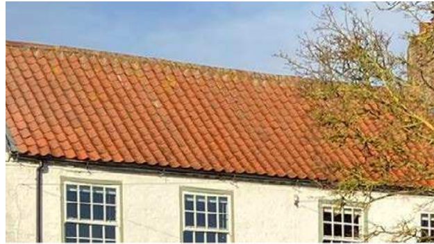
Figure 82: Red clay pantiles combined with light painted brick.
