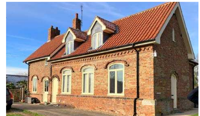
Figure 63: A 1.5 storey cottage in Searby.
