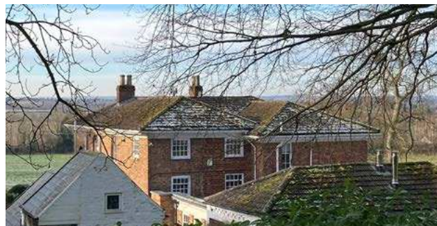
Figure 39: The Old Vicarage (Searby) (Grade II Listed). Red brick, painted ashlar dressings, tiled hipped roof with deeply overhanging plain eaves.
