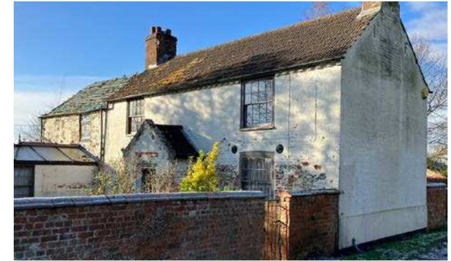
Figure 62: A two storey cottage in Owmbly.
