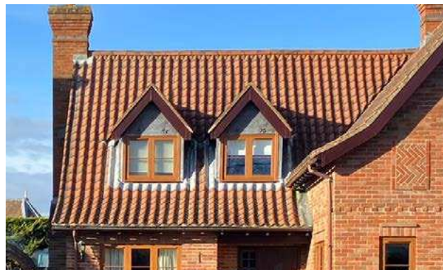
Figure 86: Modern use of red clay pantiles.
