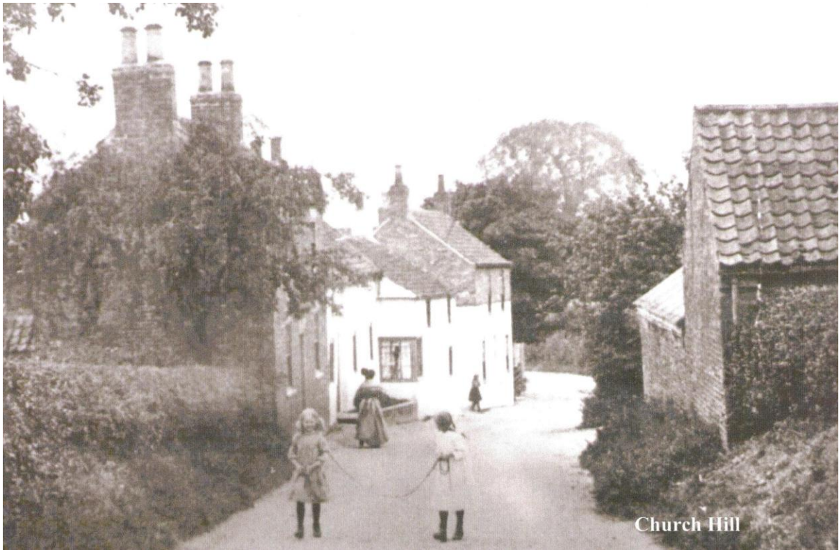
The two middle cottages on the left and the farm buildings on the right have since been demolished
