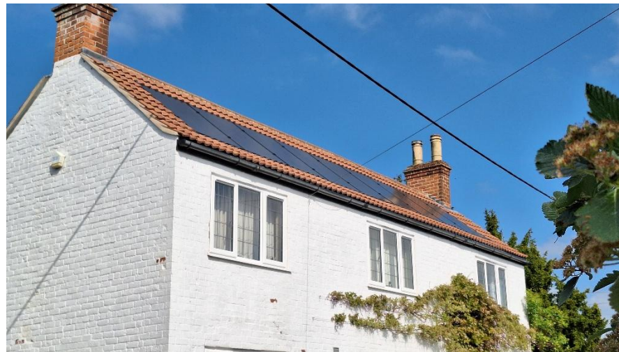
Solar panels fitted in-roof on 19 th century dwelling, Grasby
